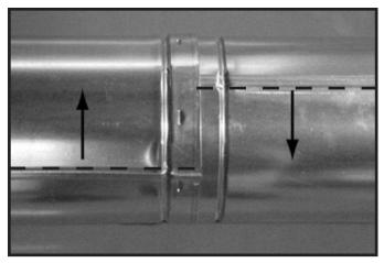
Figure 10.7 Rotate Seams for Disassembly
